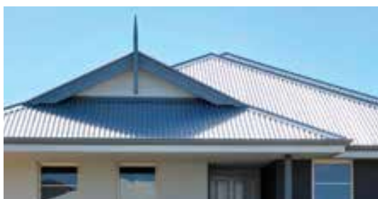
Corrugated metal deck roof
